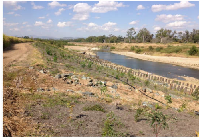
Above: O'Connell River contract revegetation site . This photo was taken in September 2019 Photo: C. Barbeler
